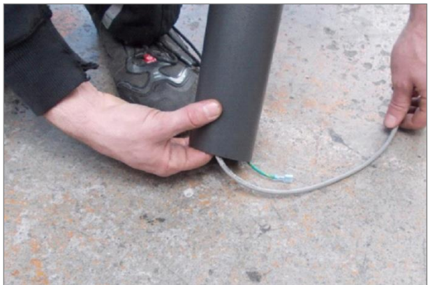
Fig. 25 Desmo assembly, wiring
